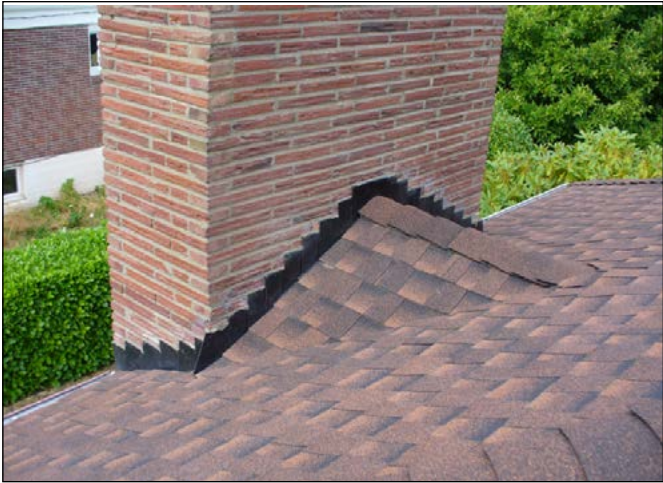
Cricket or saddle at chimney.
