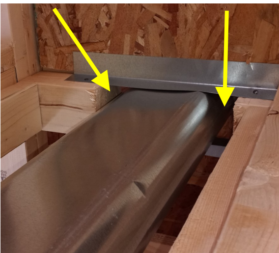
Examples of Fire Blocking needing to be added between the wall and ceiling.
